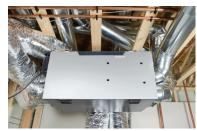
The humidistat is usually located in the hall or living room and should be set in the comfort zone or at approximately 35% to 40%. When the moisture level rises above this amount the HRV will start up and lower the level to 35% to 40%. Moist air is much more expensive to heat than dry air so there is very little cost, if any, to operate your HRV.
