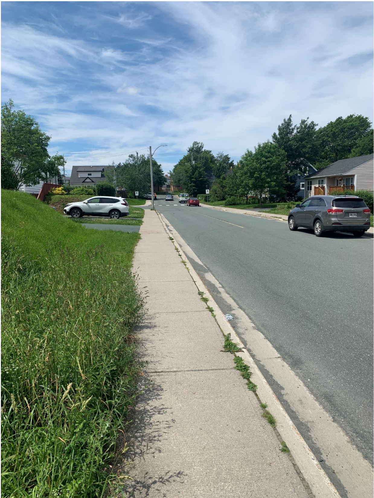
Figure 6: Site Access, Sight Line West of Access (Looking to the Left)
